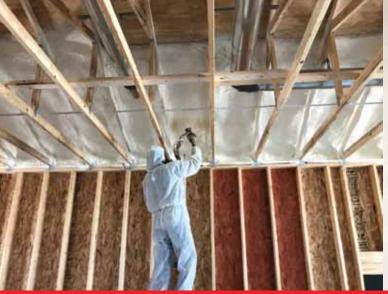
ThermoSeal Closed Cell Spray Foam creates an Air Barrier, Vapor
